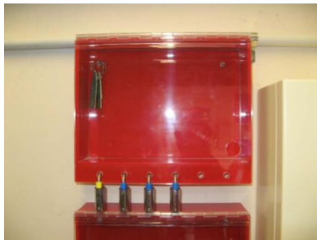
Transpower lockout box showing yellow issuer lock and blue recipient locks
