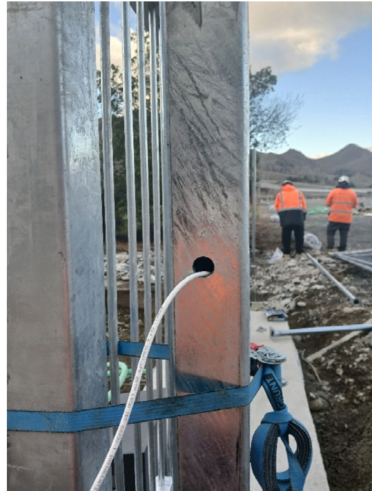
Hole drilled in post
